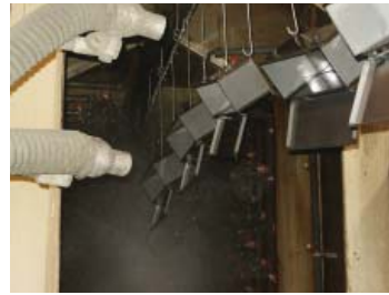
Phosphate Coating Line
