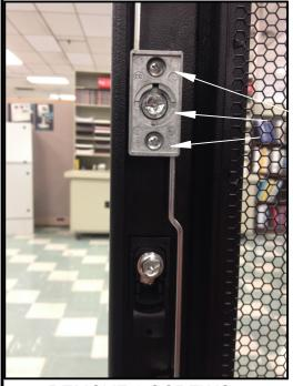
REMOVE 2 SCREWS AND RETAINING BOLT
